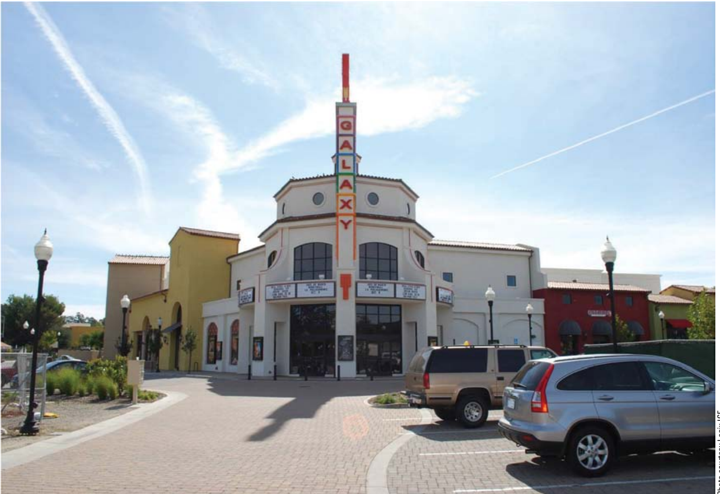
Only about one-quarter to one-eighth as much sound penetrates an ICF wall compared to wood frame, making them popular for movie theaters, such as this one in California's Central Valley.
