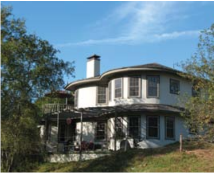
Radius walls, such as those on the Massachusetts home above, are much simpler to build with ICFs than any other construction method.
