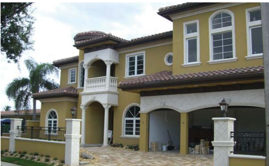
Photo courtesy Safe Harbor Design/Build
