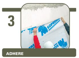
the top edge of the COLPHENE ICF membrane, making sure the membrane is well aligned.
