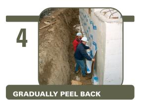
the remaining silicone release film, making sure the membrane is completely adhered.
