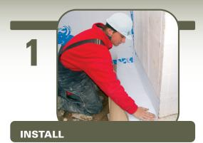
the footing membrane first, making sure that the inside corner is completely adhered.
