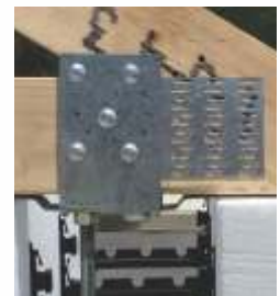
After concrete pour and set, screw truss/rafter to BHBCON
